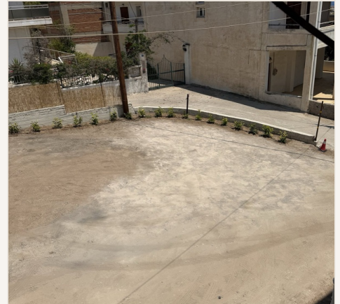
P1 — the alley beside the hotel.
